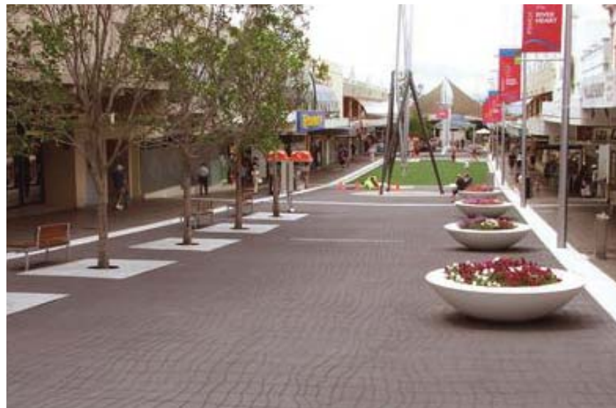
Pedestrian Area: Convert portion of parking area to pedestrian area with trees, planters and walking surfaces. Above surface is paint coating.
