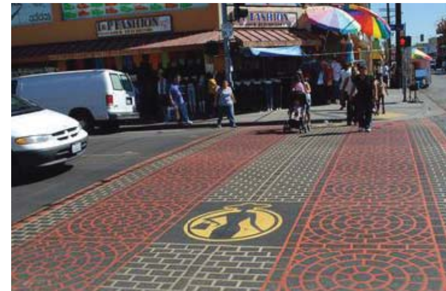
Improved Crosswalks: Clearly established crosswalks can improve pedestrian movement. Low-cost painted patterns are in increasing use.
