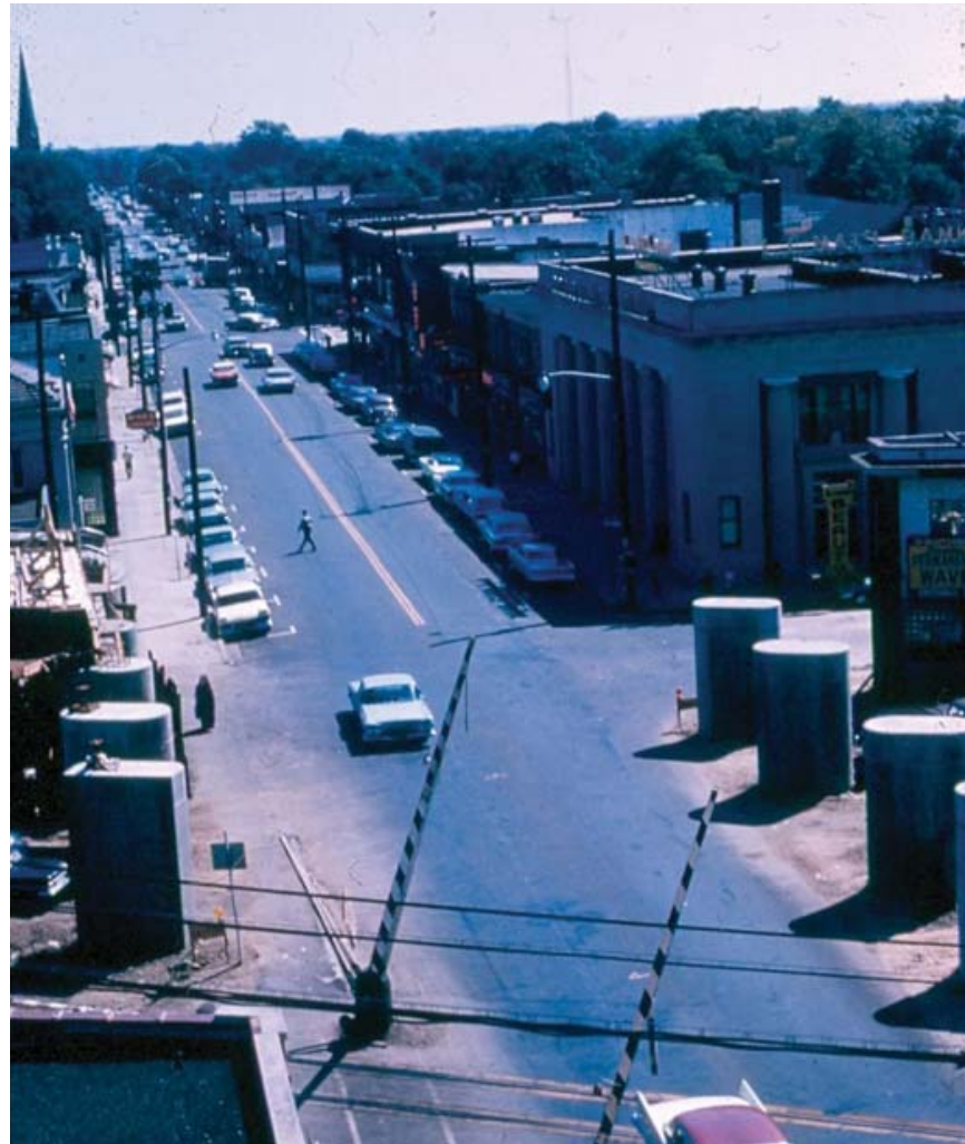
Construction of the elevated train tracks in 1963
