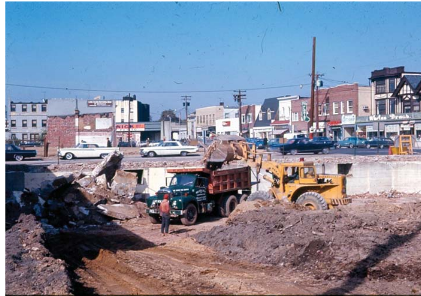
Demolition of the west side of Broadway
