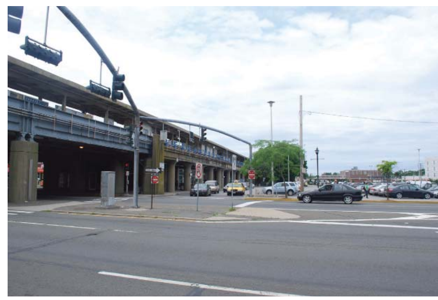
Few Crosswalks: Some of the challenges for pedestrians are streets that are difficult to cross.
