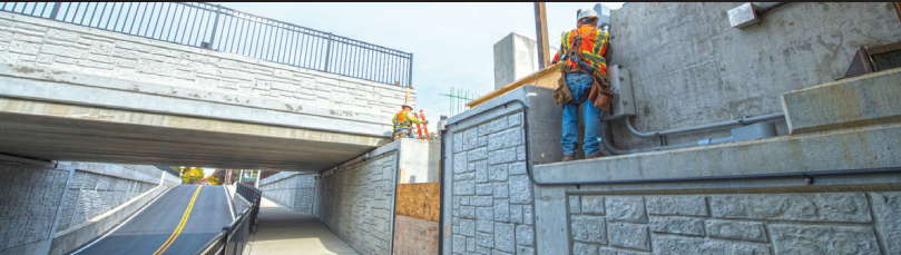
MTA-LIRR Third Track
